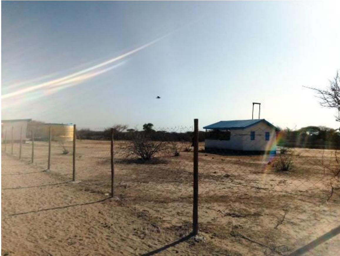
Picture showing the existing Lagdima community borehole (depth 270M, Yield 24M 3 /hr)
