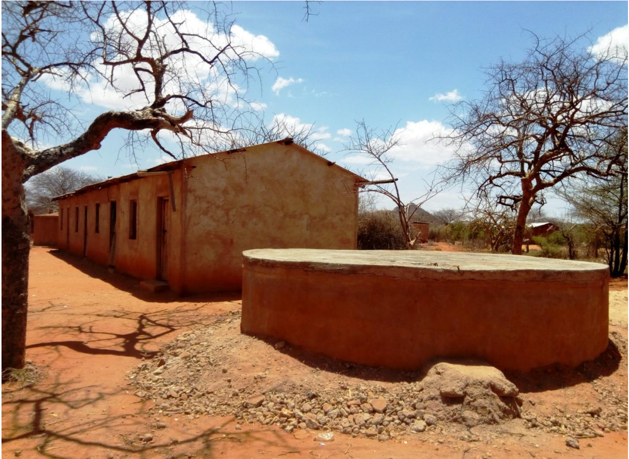
Fig.5.0: Picture showing an underground tank constructed within the school compound for water storage.
