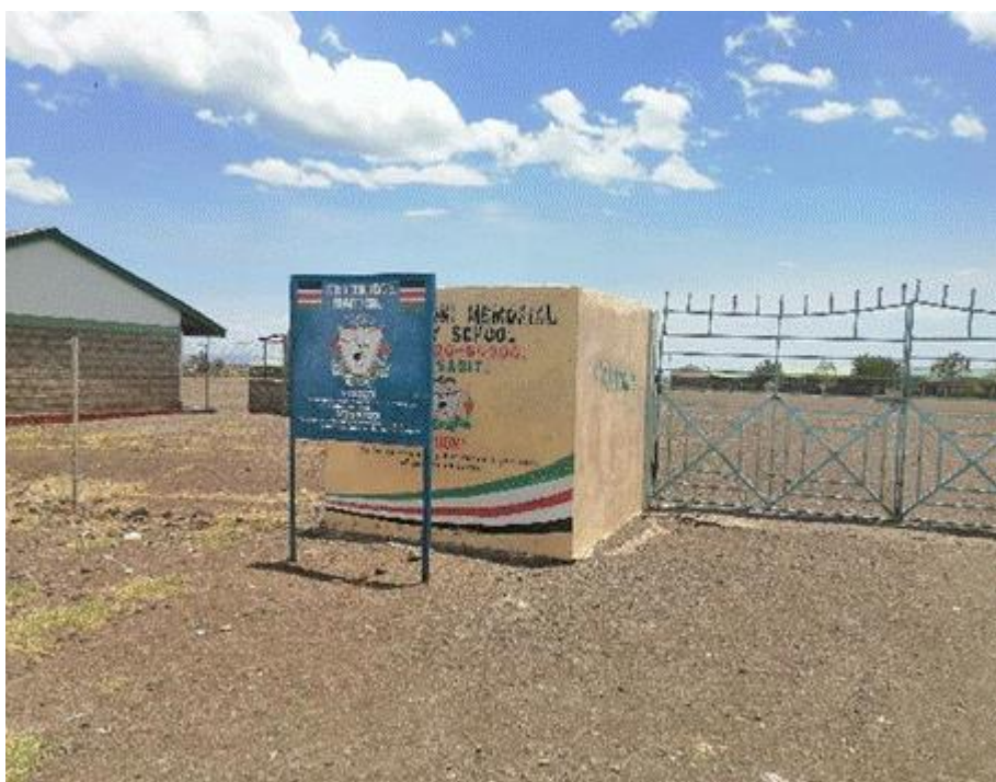
Figure 5.6: Photograph of Ngoyoni Primary School
