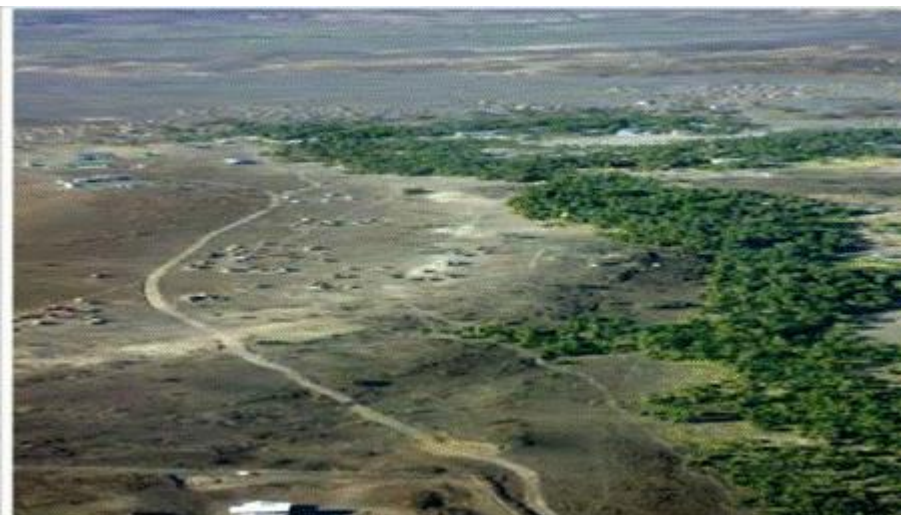
Figure 5.3: Photographs of Road Infrastructure
